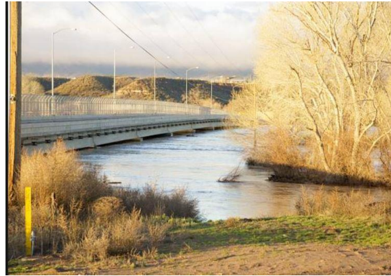
Figure 1.2: Flooding on Duncan Bridge (2005)
